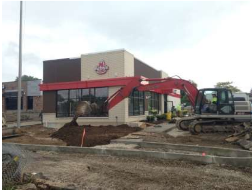
Photograph A: Existing Arby's Signage per Permit (Wall Sign and Side Entry Door "Arby's")
