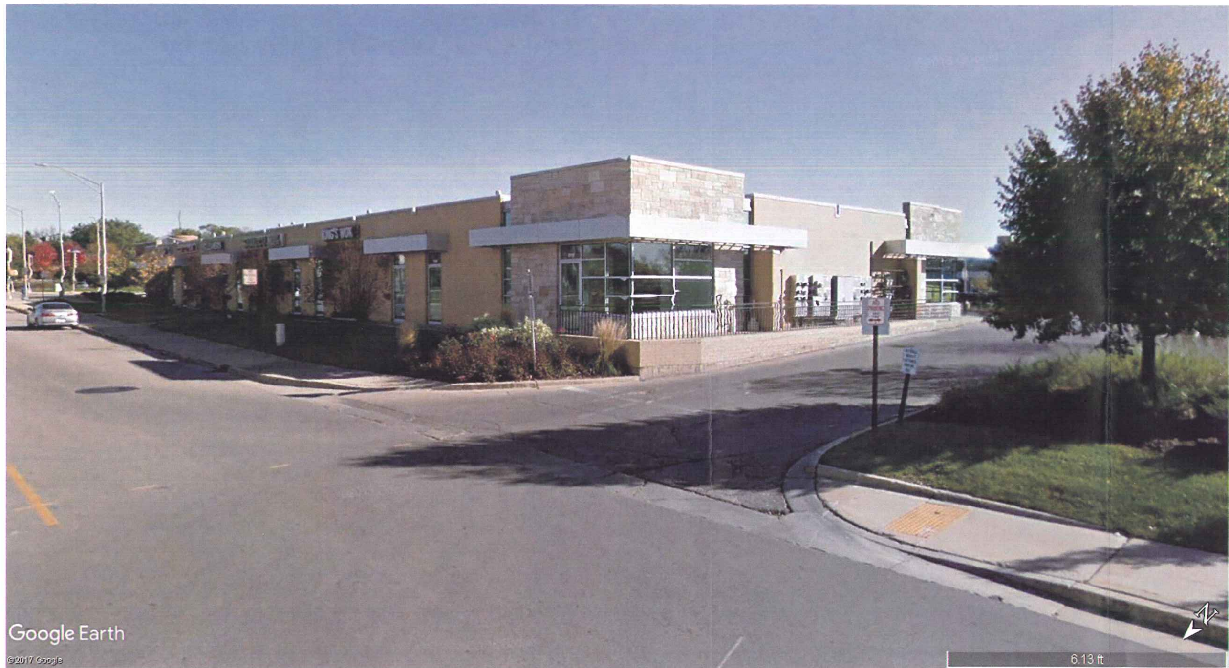
1 EXISTING EXTERIOR STREET ELEVATION
