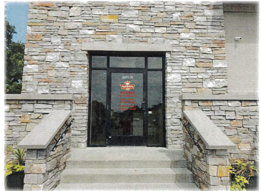
New Graphics in Place
