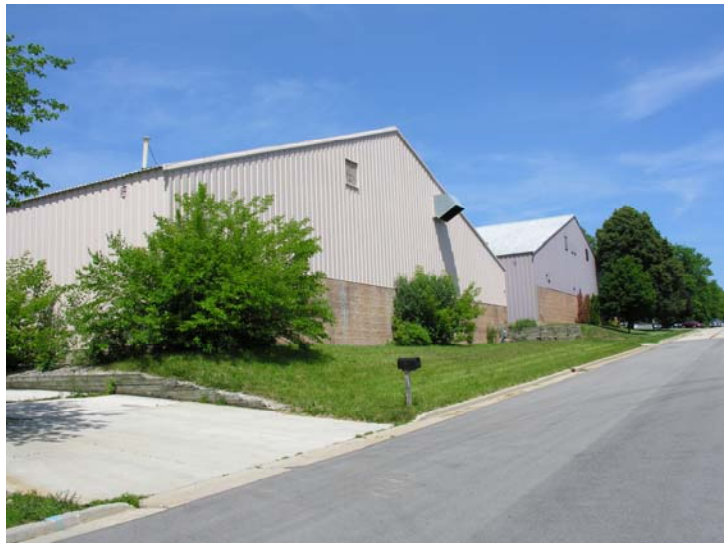
Photograph 1. View from the southwest of 2920 (left) and 2916 (right) West Vera Avenue. 2916 is occupied by the Paley Tennis facility.
