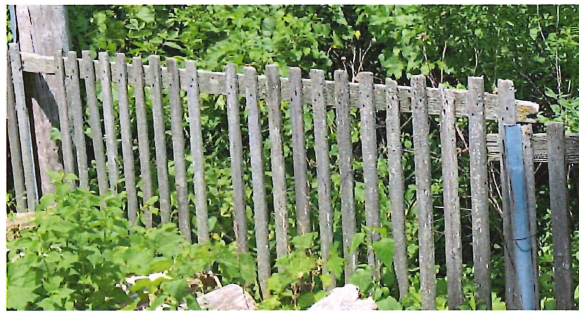
Broken Fence Taking Down
