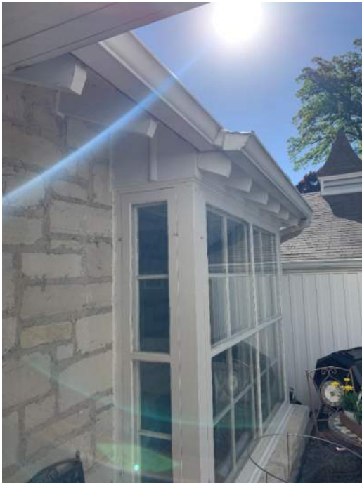
Existing Rafter Tail Details at Front Elevation
